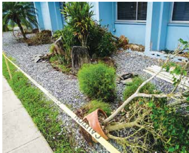
Landscaping work started around the Administration building (in picture shown), also around the Canteen, Safety, Technical Buildings and Warehouse.
