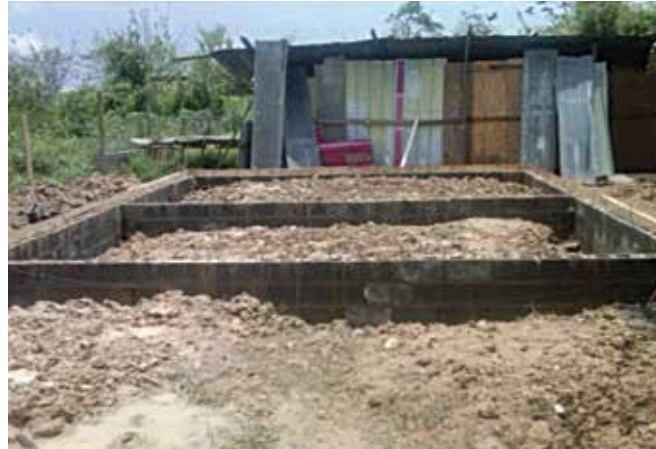
Foundation of the Singh's home with the old home behind.
