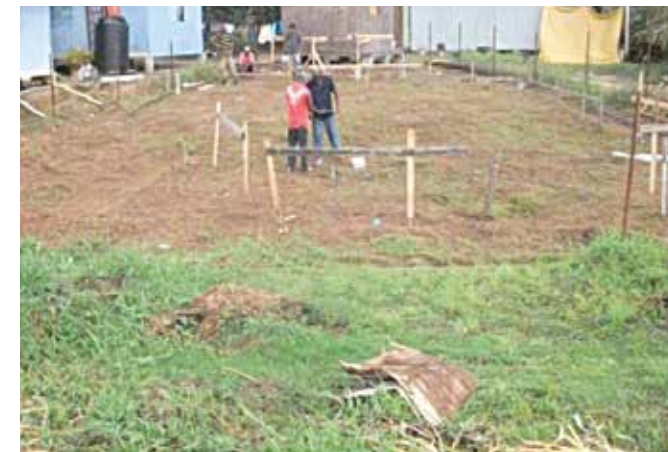
Site preparation for Cecelia Small's foundation
